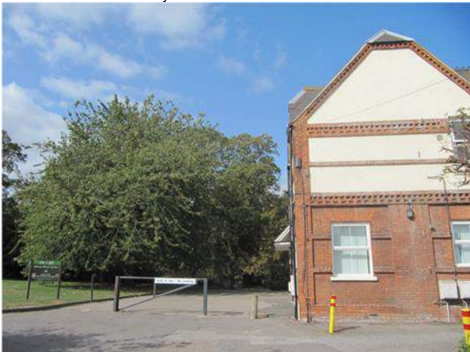
Main entrance from Burley Road showing Old Johnson house
